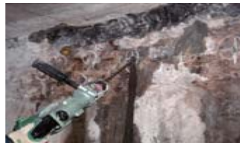
Salt damage prevention work
