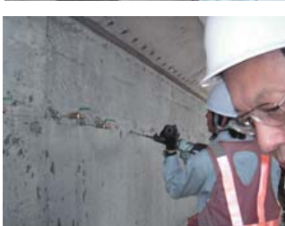
JR Tokai - Shinkansen bridge piers deterioration prevention and leakage repair work
