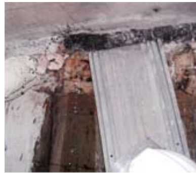
There are more than 20 liters of water leakage per minute from this area
