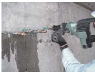
Nursing home bathtub leak repair waterproof construction
