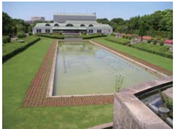
Water leak repair waterproof construction of fountain pond park
