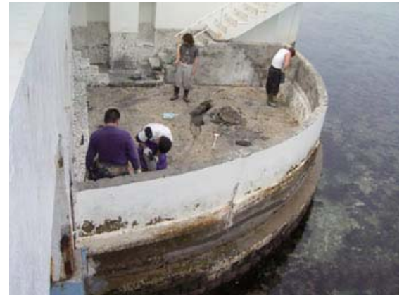
Refurbishment of the swimming pool which opened to the ocean Waterproof construction
